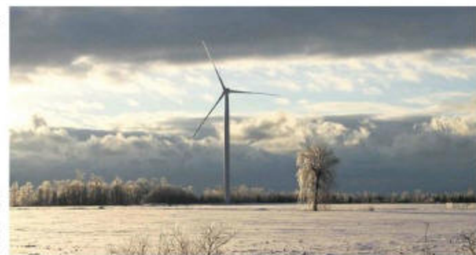
LEADING THE FIELD: One of the six Vestas V82-1.65MW turbines at the Frogmore wind farm, Ontario
